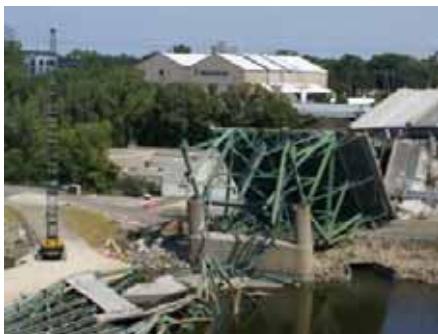
Figure A: I-35W Bridge Following Collapse in Minneapolis, MN
